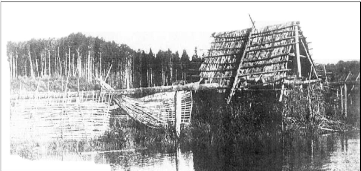
Figure 3.4. Smokehouse where the fish are hung during the first stage of processing. Roof is constructed from spruce bark.
