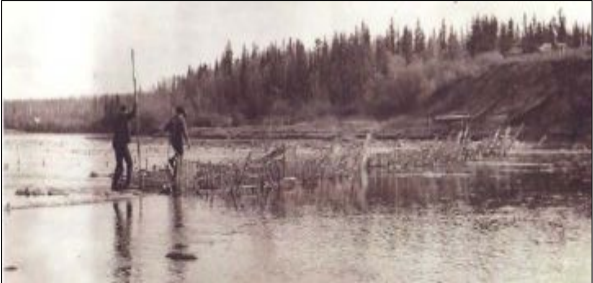
Figure 3.3. Salmon weir at Fraser Lake October 1903.
