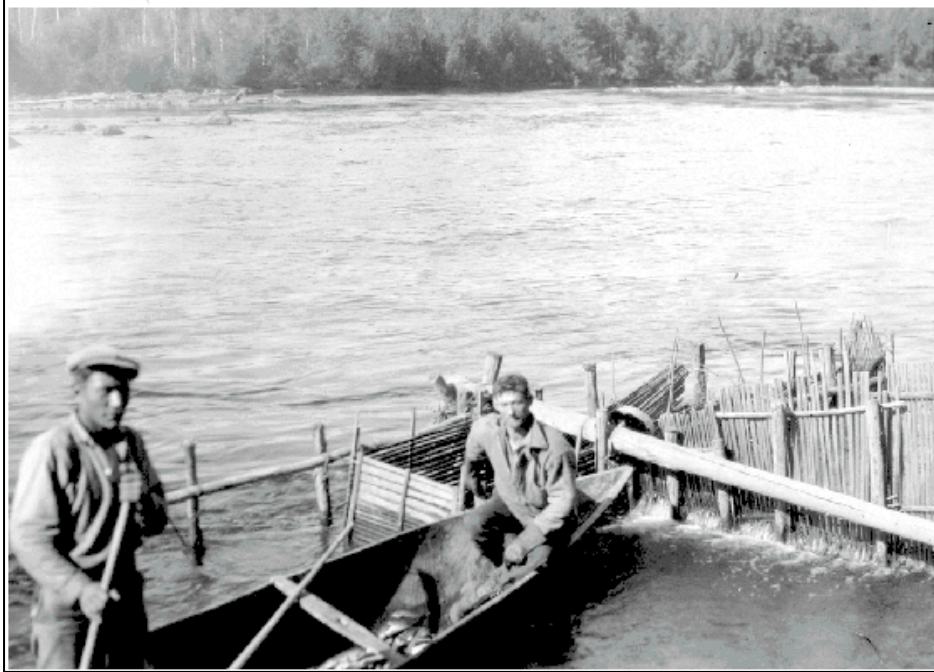
Figure 3.8. Partial weir and fish trap known as a koonsai for fishing kokanee on the Tachie River.
